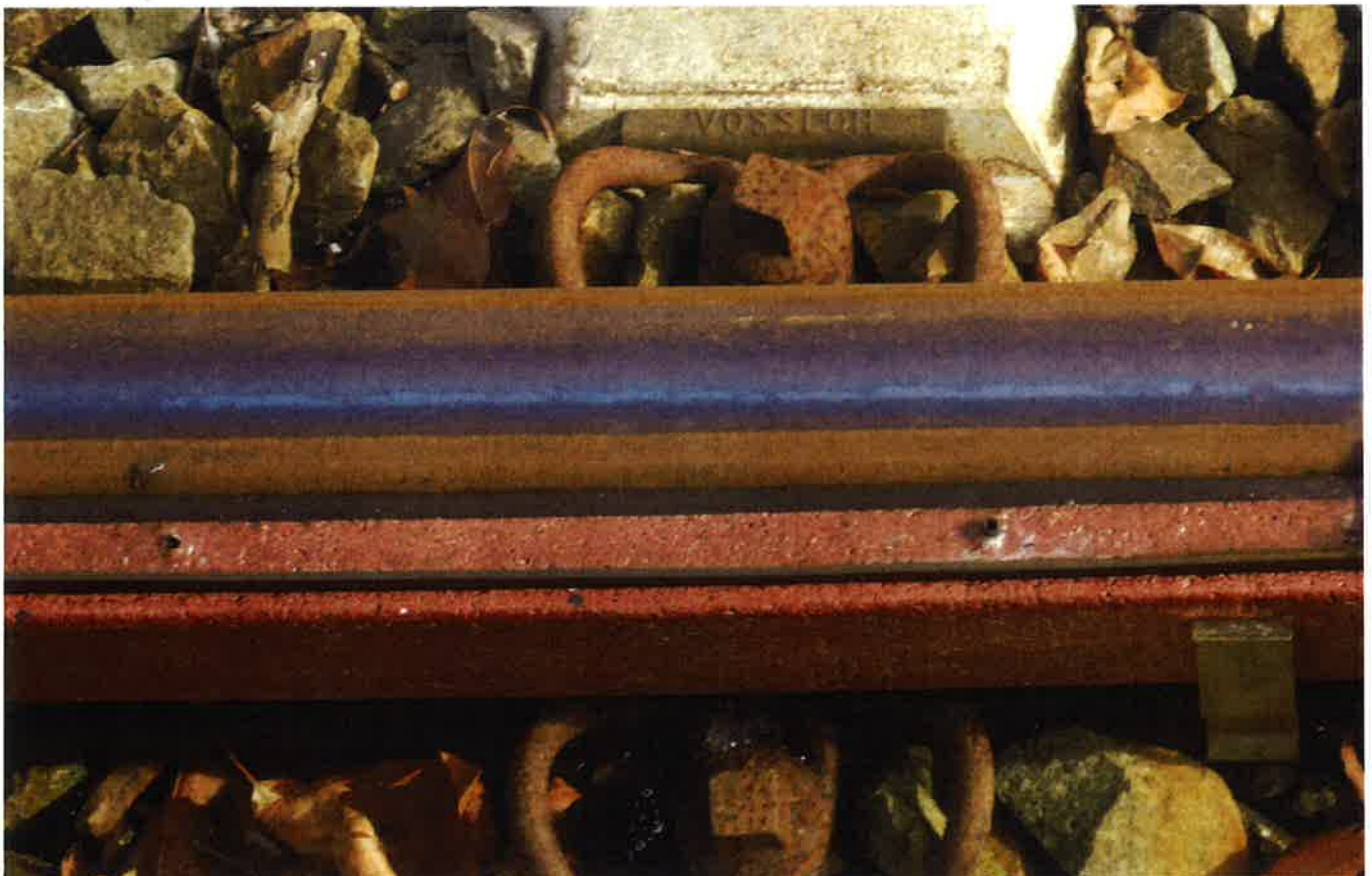
The WSI's running surface, dripping tube and limiting strip fits seamlessly with the rail profile.
